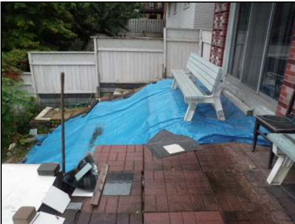
Figure 7. Active erosion in the rear yard at No. 43 Troutbrooke Drive. Source: TRCA, 2010.
