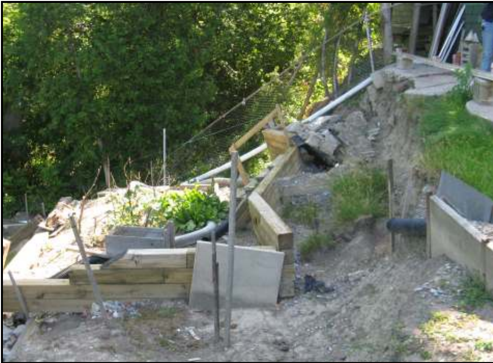
Figure 6. Failed retaining walls in the rear yard at No. 51 Troutbrooke Drive. Source: TRCA, 2009.
