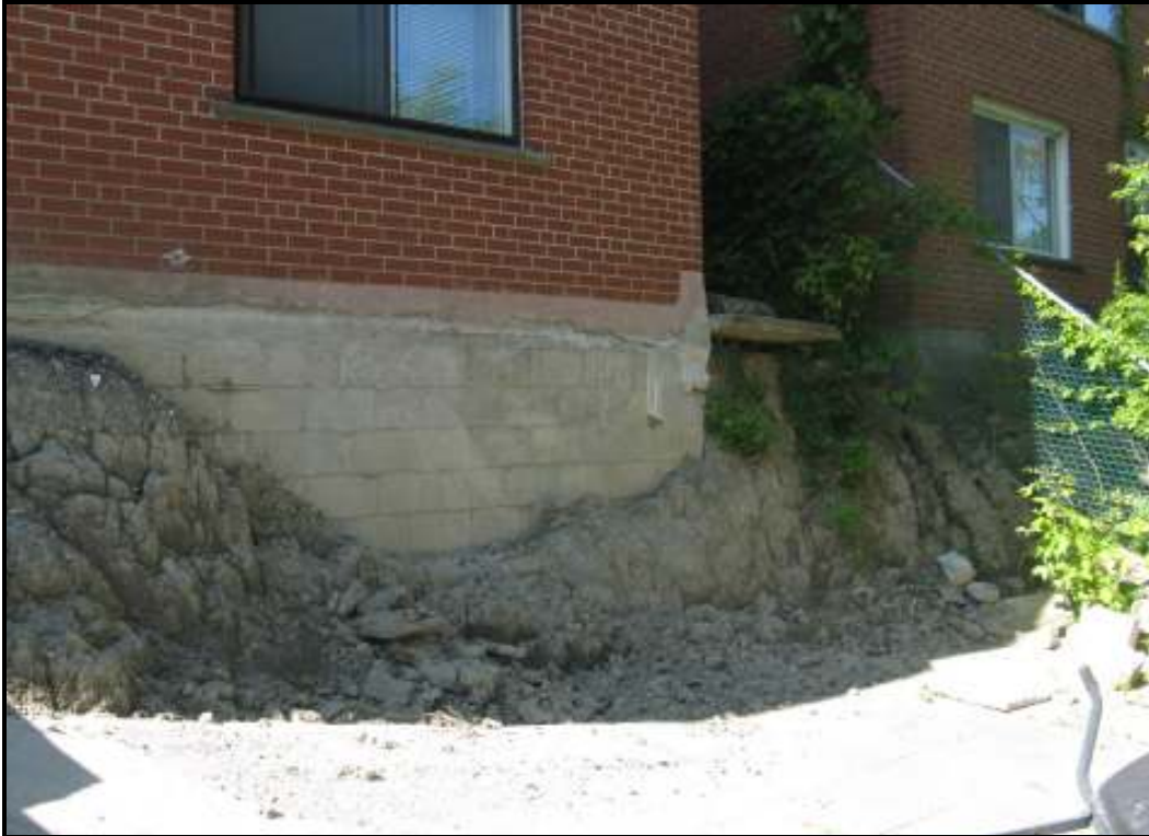
Figure 4. Active erosion exposed foundation at No. 45 Troutbrooke Drive. Source: TRCA, 2009.
