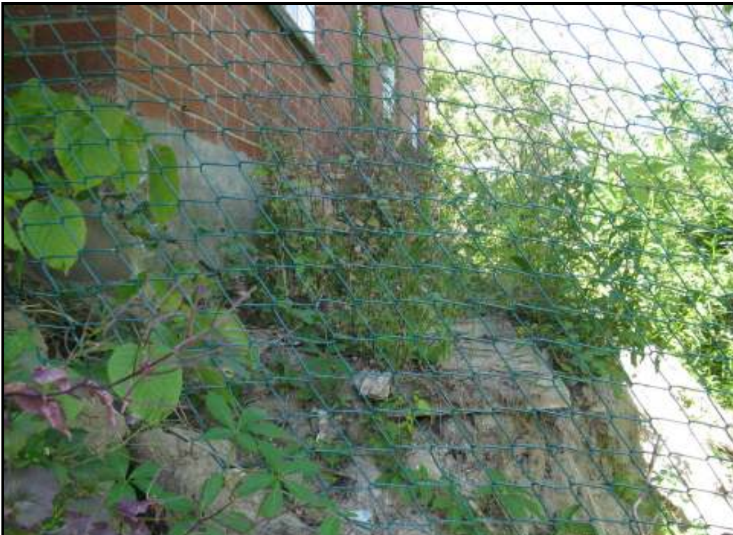
Figure 5. Active erosion exposing foundation at No. 47 Troutbrooke Drive. Source: TRCA, 2009.
