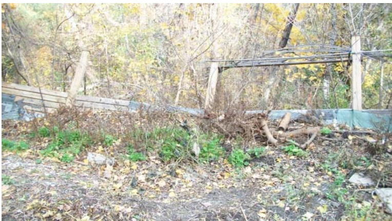
PHOTOGRAPH No.18 Slope face directly north of 45 Troutbrooke Dr., failed retaining wall, looking north.
