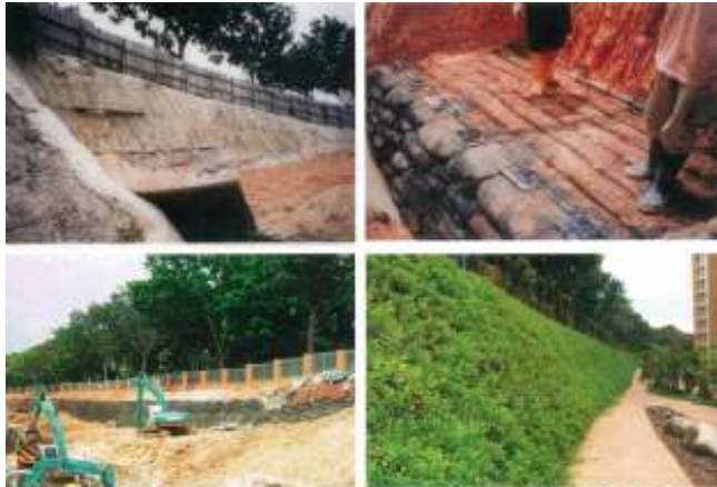
Green Retaining Wall
