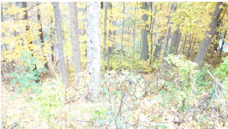
PHOTOGRAPH No.12 Slope face directly north of 41 Troutbrooke Dr., well vegetated, looking north.
