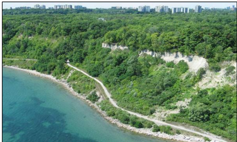
Existing access road below Guild Inn/Guildwood Parkway.
