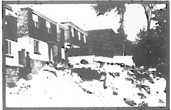
IMPROPER CONSTRUCTION PRACTICES RESULTED IN BANK FAILURE WHICH SEVERELY THREATENED THESE HOMES
