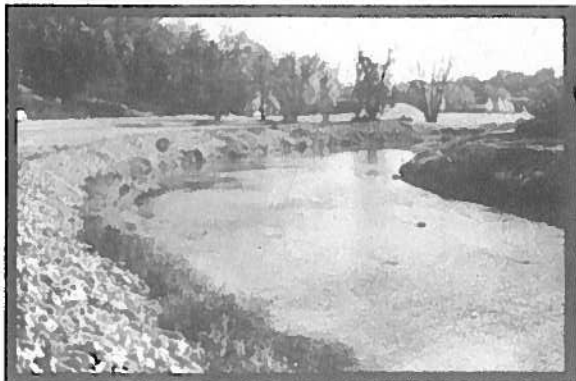
RIP RAP (PHOTO 18)
